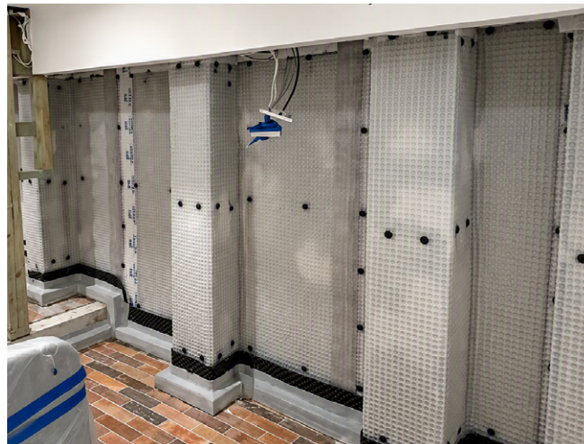
Pic 6. Negative-side waterproofing – Newton 503 Cavity Drain Membrane System used for an internal remedial application.
