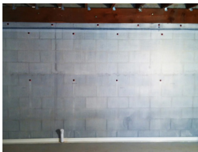
Pic 7. Negative-side waterproofing – Newton System 500 cavity drain system installed for an internal remedial application.
