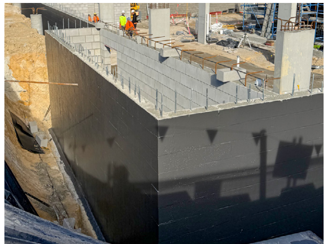
Pic 4. Positive-side waterproofing – WPA waterproofing system comprising WPA 560, WPA 992.
