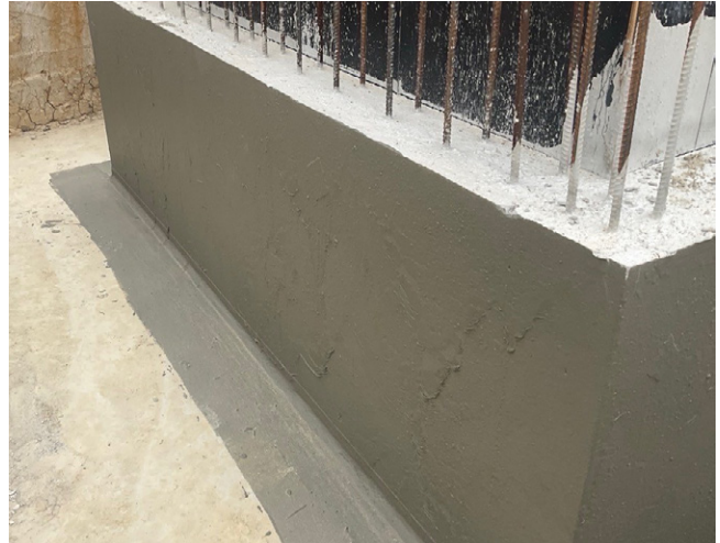
Pic 3. Positive-side waterproofing applied during new construction.
