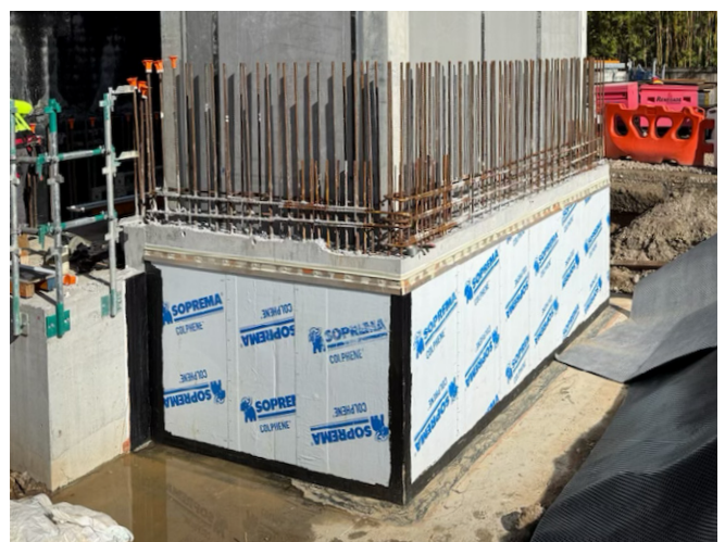
Pic 5. Positive-side waterproofing – Soprema Colphene 3000 System installed to a lift fit.
