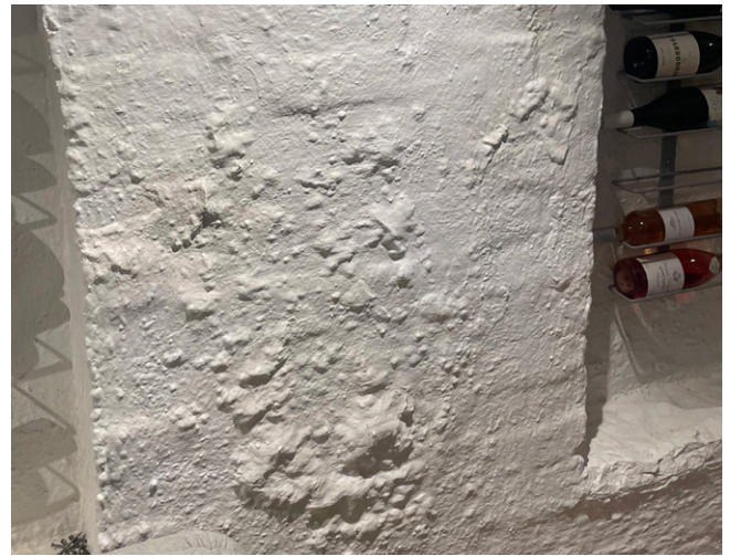
Pic 2. Existing substrate conditions prior to installation of the Newton cavity drain system.
