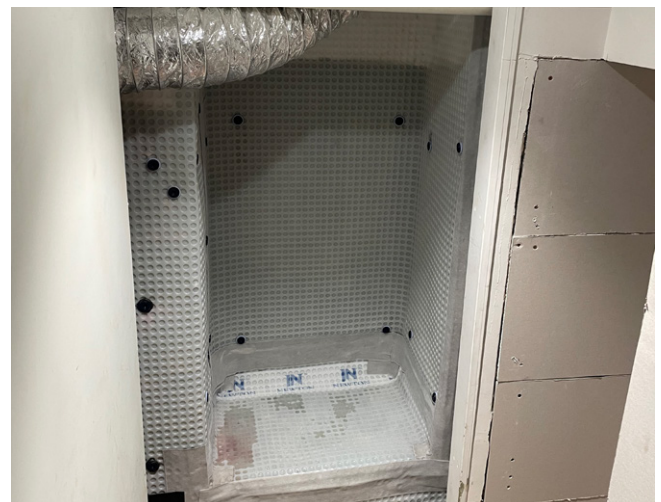
Pic 3. Newton 503 Cavity Drain Membrane System installed to manage groundwater ingress.
