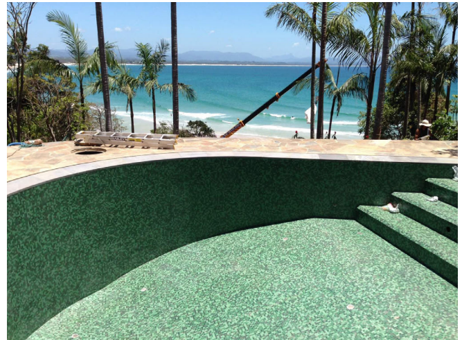
Pic 6. A good example of pool waterproofing using the LATICRETE Pool System.
