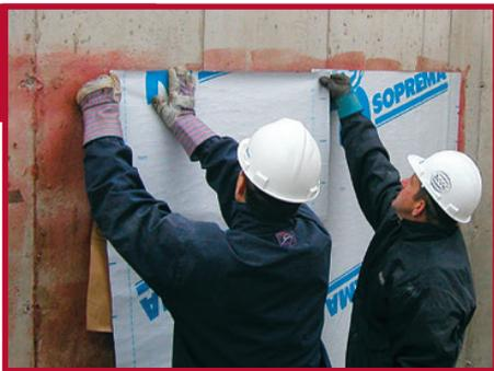
Peel back the top part of the silicone release film. Adhere COLPHENE 3000 to the substrate, making sure the membrane is well aligned.
