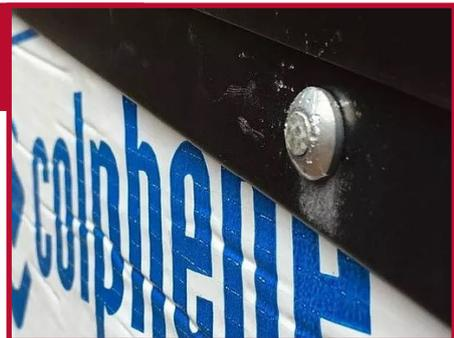
Use a pressure seal termination barre with a bead of SOPRAMASTIC / SOPRAMASTIC ALU to seal the membrane termination.
