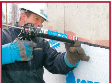
Use SOPRAMASTIC / SOPRAMASTIC ALU to seal details and critical areas.
