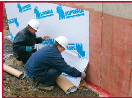
Gradually peel back the remaining silicone release film, making sure the membrane is completely adhered.
