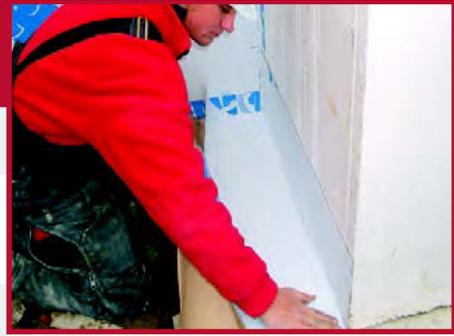
Install a reinforcement strip membrane centered on the corner of all interior and exterior foundation angles.
