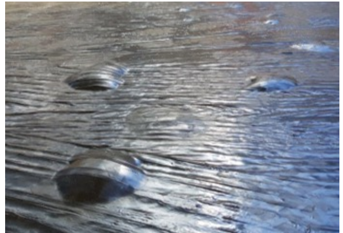
1. Blistering of membrane due to entrapped moisture
