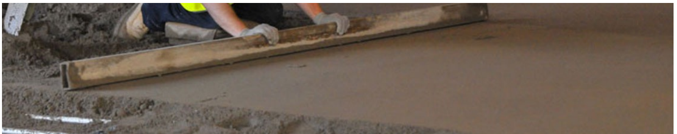
Take note of the thickness and consistency of the screed
