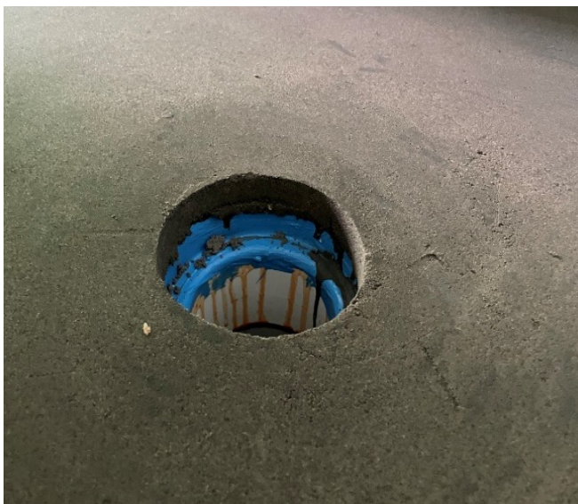
Screed to drainage flange is ready for waterproofing
