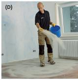
To accelerate the setting proces, up to max. 4% of UZIN Epoxy Accelerator can be added to the primer. The application of the following coat can therefore be carried out earlier, ideally at the same day.
