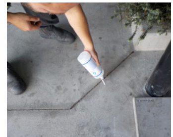
4. Pour into crack and allow to dry before overcoating.
