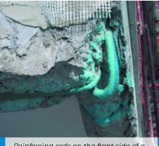
Reinforcing rods on the front side of a balcony treated with Mapefer 1K
