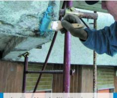
Applying Mapefer 1K with a brush on reinforcing rods on a reinforced concrete balcony
